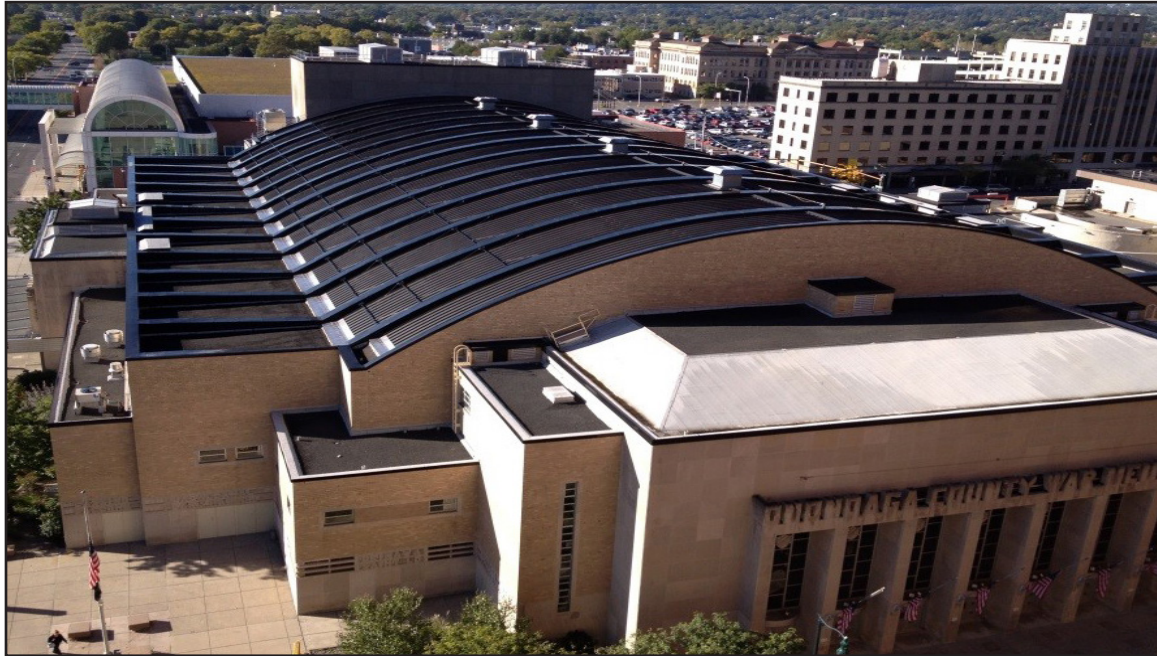
Aerial of new roof
