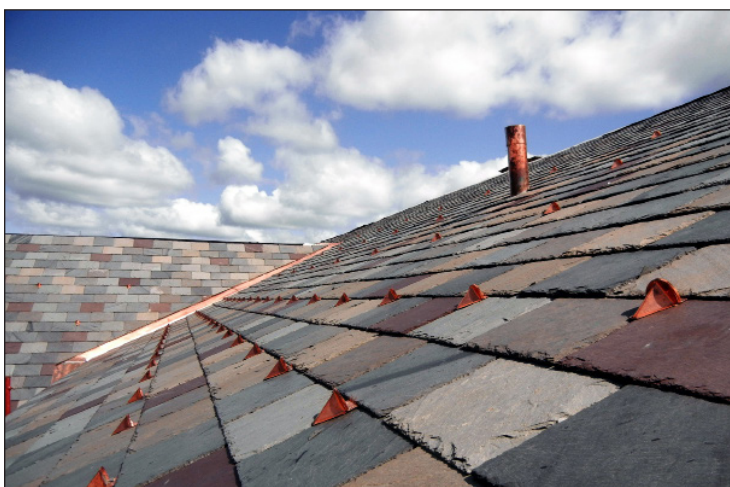
Slate Roofing, Historic Preservation
