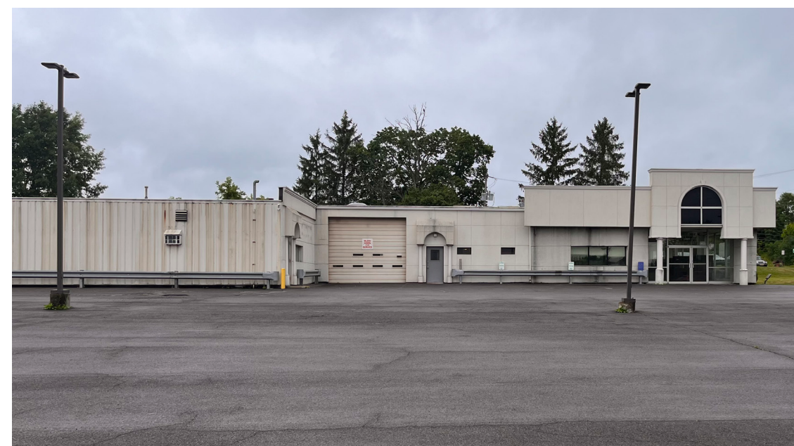
BUILDING A EXISTING PHOTO SOUTH
