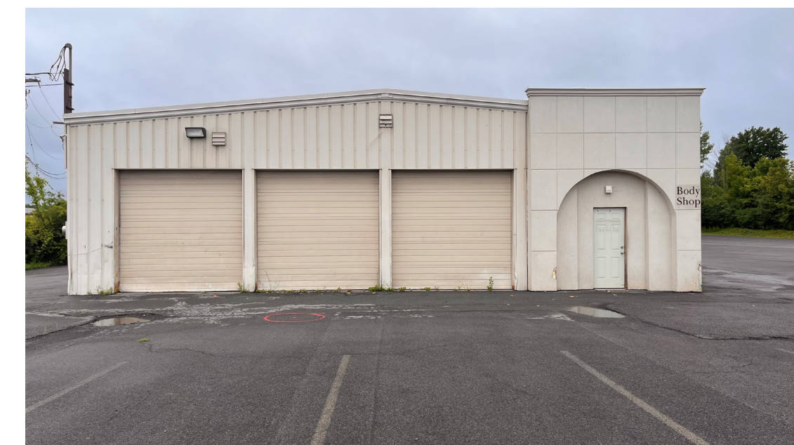
BUILDING C EXISTING PHOTO EAST
