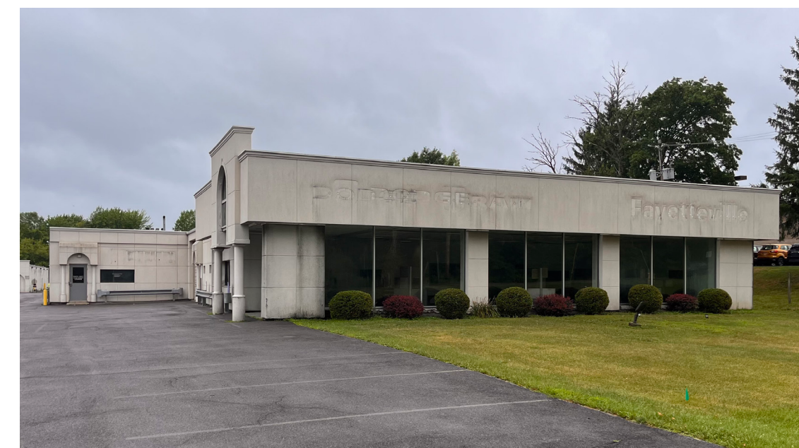
BUILDING A EXISTING PHOTO EAST
