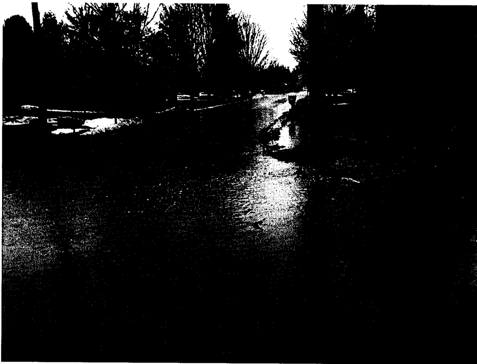
Intersection of Muirfield Drive w/ Hoag Lane, note all catch basins are surcharged 1/12/18
